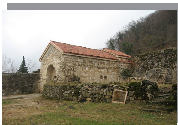
Gelati. Entrance gate after restoration, 2010
