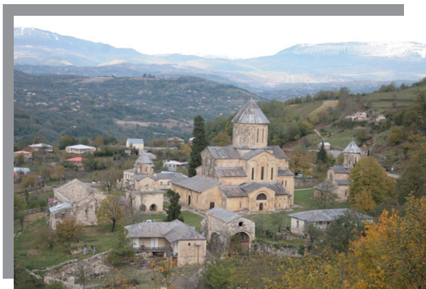
Gelati before restoration, 2007
