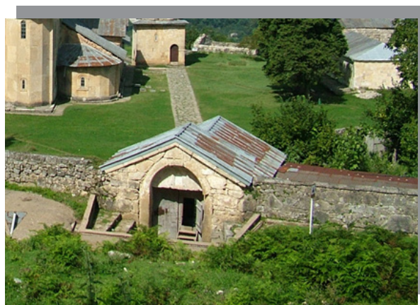
Gelati. Entrance gate before restoration, 2009
