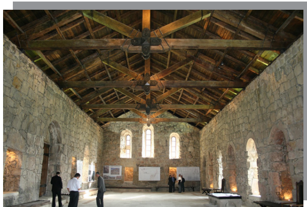
Gelati Academy after restoration, 2009
