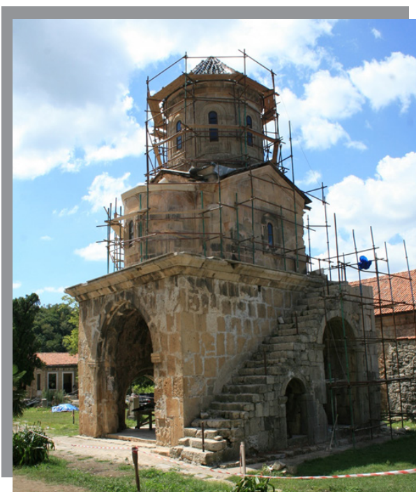
Gelati. St. Nicholas Church under restoration, 2011
