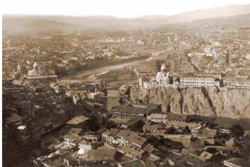
Tbilisi. A royal palace used to stand next to Metekhi church.
